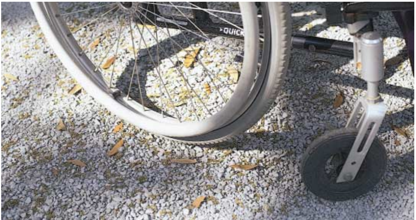
Wallace Residence, Savannah, GA—Gravelpave 2 creates a wheelchair-accessible surface by stabilizing gravel and supporting tire pressure. 7% dry cement was mixed with gravel before filling rings. Cover photo: Westin Kierland Resort and Spa, Scottsdale, Arizona—Grasspave 2 fire lane and Gravelpave 2 fire lane (concrete widening).
