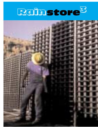
Rainstore³ is the new standard in efficient sub-surface stormwater storage. Rainstore³ is modular and stackable for versatile site design. Rainstore³ is 94% void space and can be designed for detention, retention, or water harvesting for re-use.
