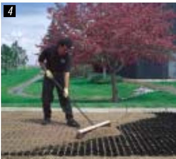
4 Fill rings with clean sharp concrete sand.
