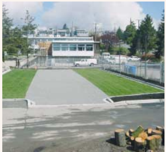
City of White Rock Operations, White Rock, British Columbia—Gravelpave 2 is used in the main drive aisle of the works yard and Grasspave 2 is used for the parking bays.
